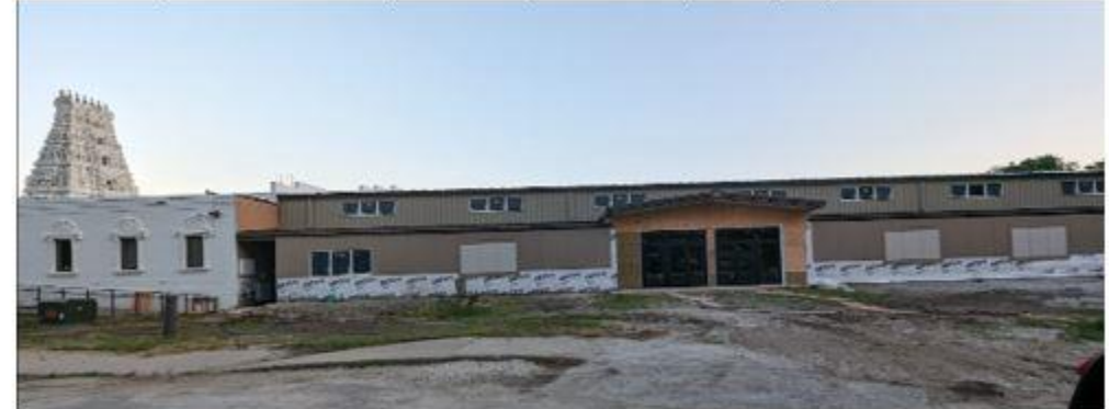
North exterior; interior wall framing; mechanical, electrical and plumbing rough-in started
